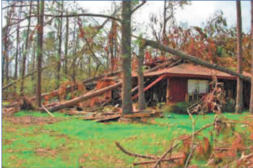
FIGURE 4-23: A home damaged by fallen trees during Hurricane Katrina (Diamondhead, MS) (SOURCE: FEMA 549)
