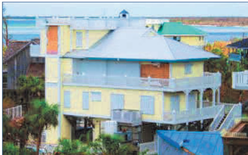
FIGURE 2-3: Building built to the 2001 Florida Building Code (FBC) standards with no structural damage after Hurricane Charley (North Captiva Island, 2004) (SOURCE: FEMA 488)
